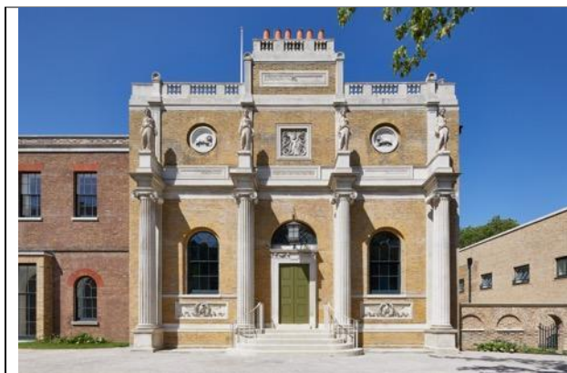
Front façade of Pitzhanger Manor. © Pitzhanger Manor & Gallery. Photo by Andy Stagg
